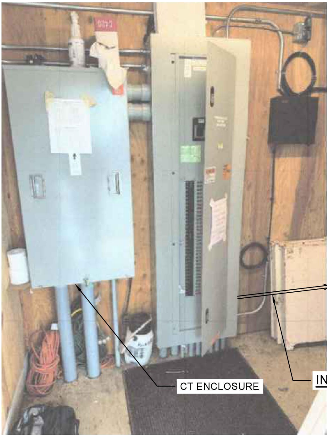
EXISTING PANEL AND METERING N.T.S
