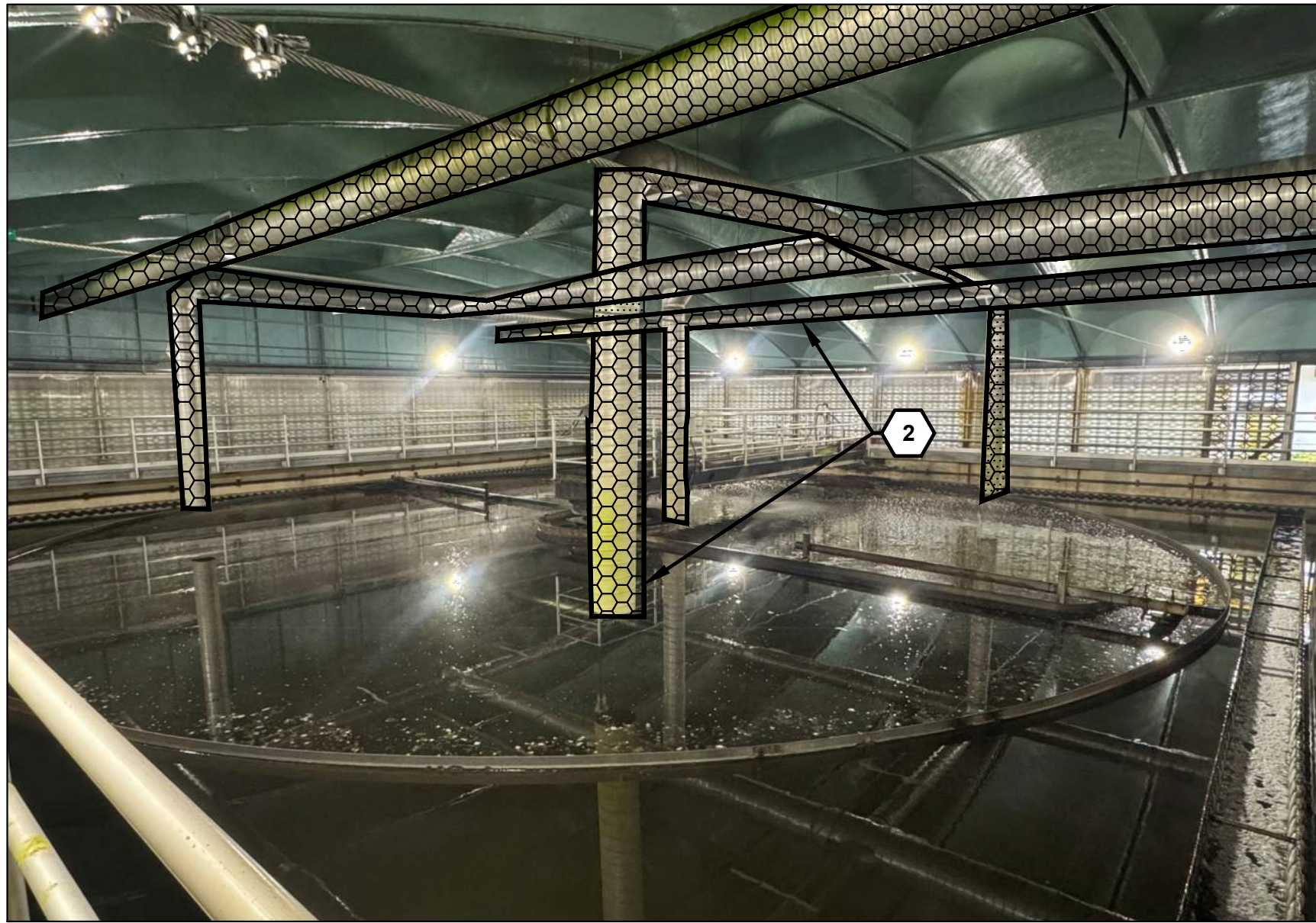
3 SECONDARY CLARIFIER FOUL AIR DUCTING (TYP)
