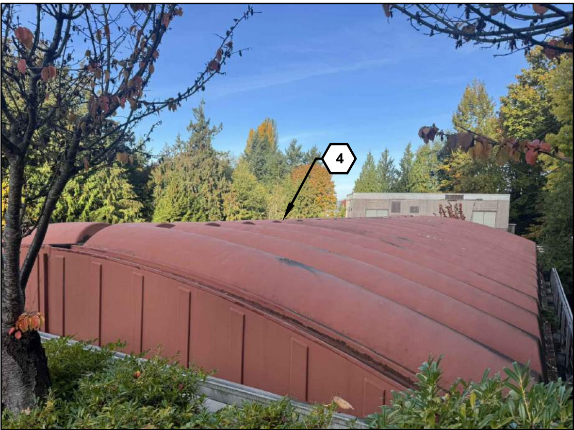
2 SECONDARY CLARIFIER BUILDING G-08 EXISTING CONDITIONS
