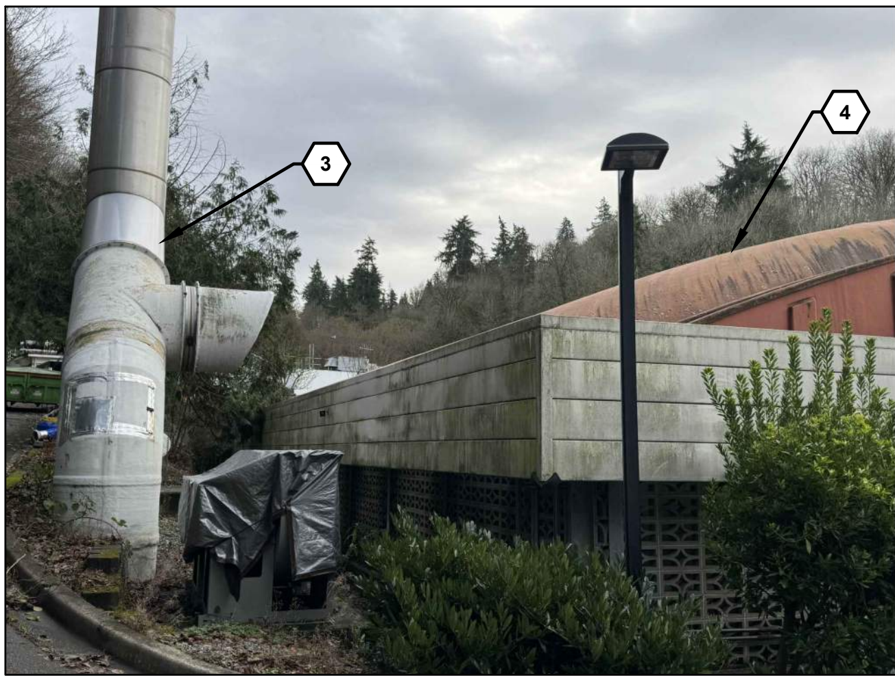
5 SECONDARY CLARIFIER BUILDING G-08 FOUL AIR EXHAUST STACK EXISTING CONDITIONS
