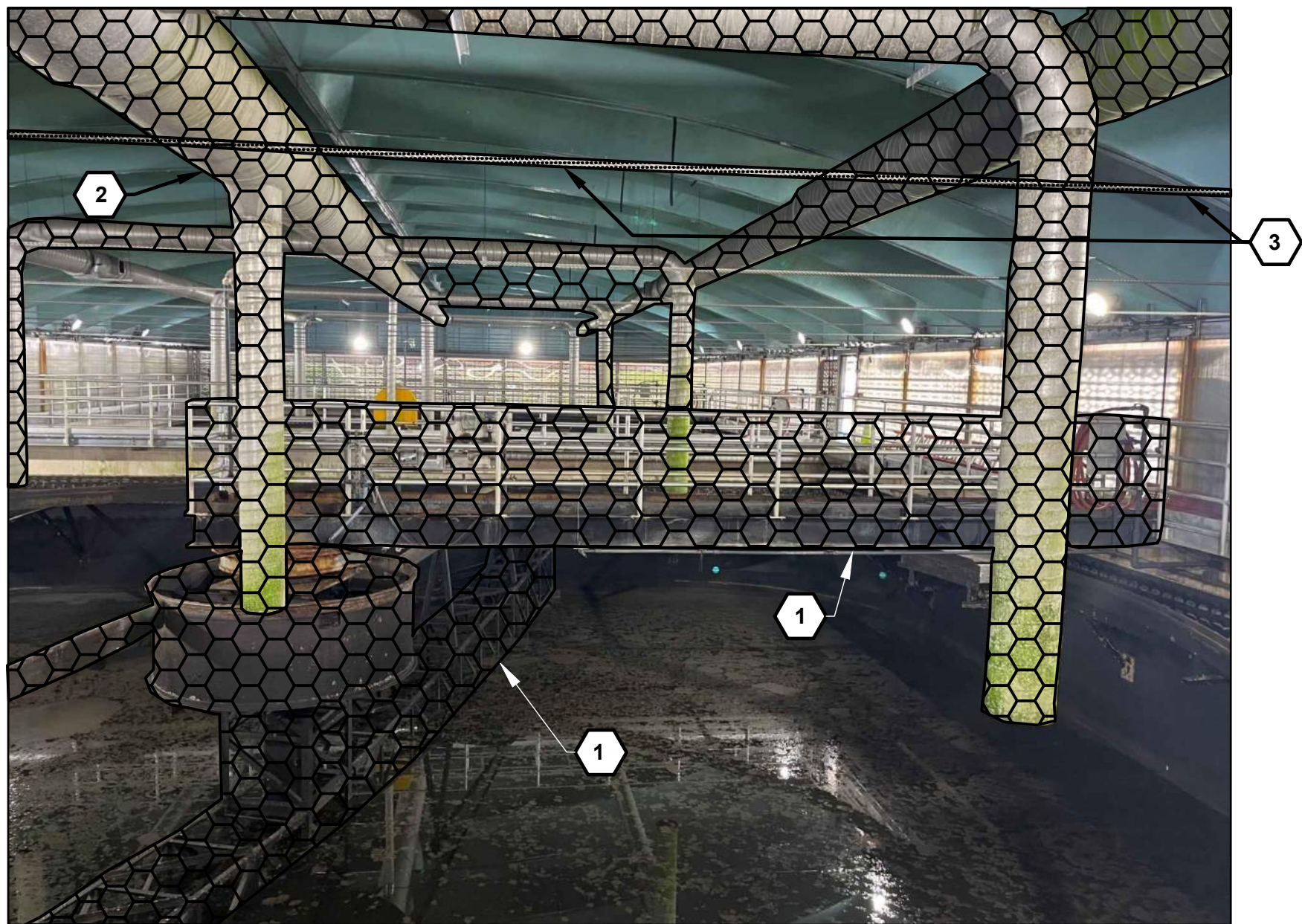
4 SECONDARY CLARIFIER RAKE ARM AND PLATFORM (TYP)
