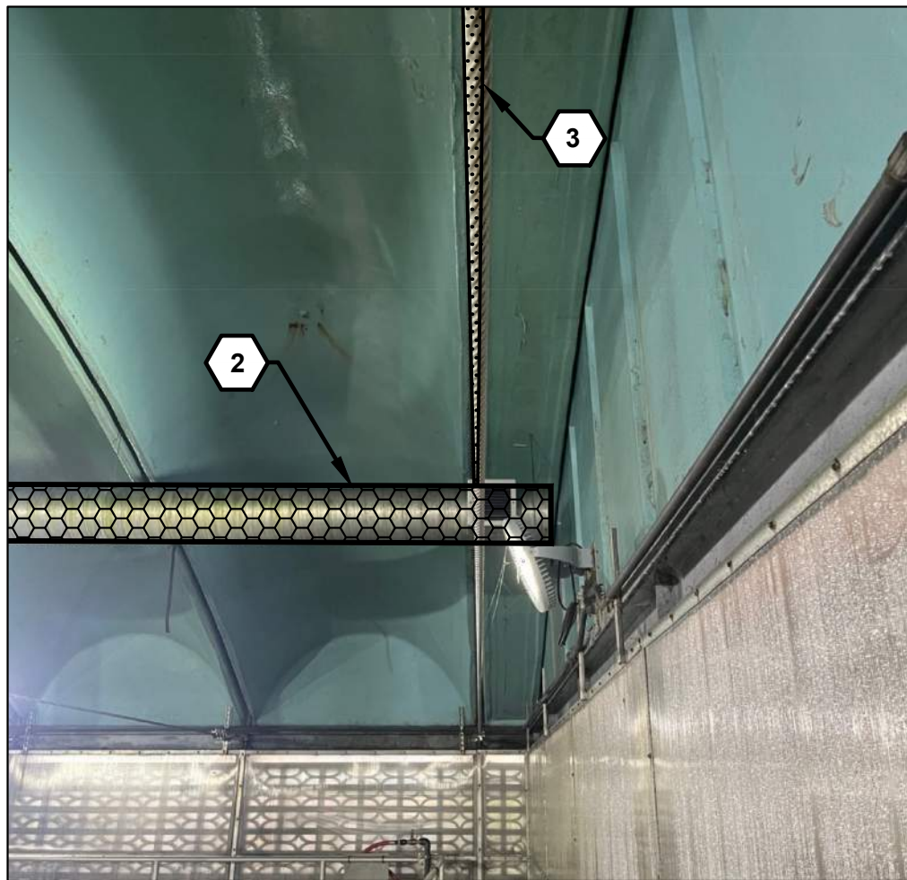
5 SECONDARY CLARIFIER FOUL AIR DUCTING (TYP)
