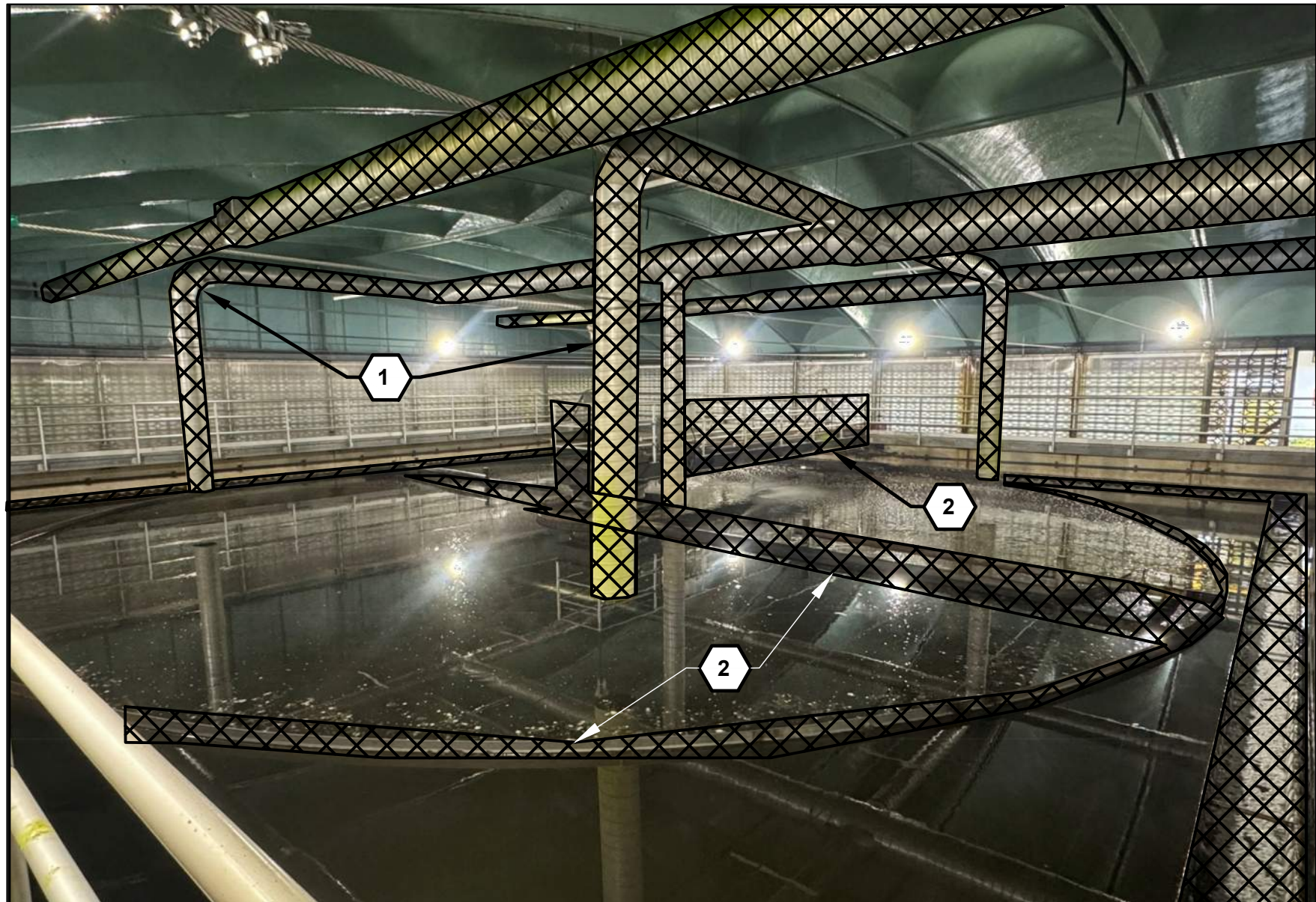
3 SECONDARY CLARIFIER D-04 FOUL AIR DUCTING (TYP)
