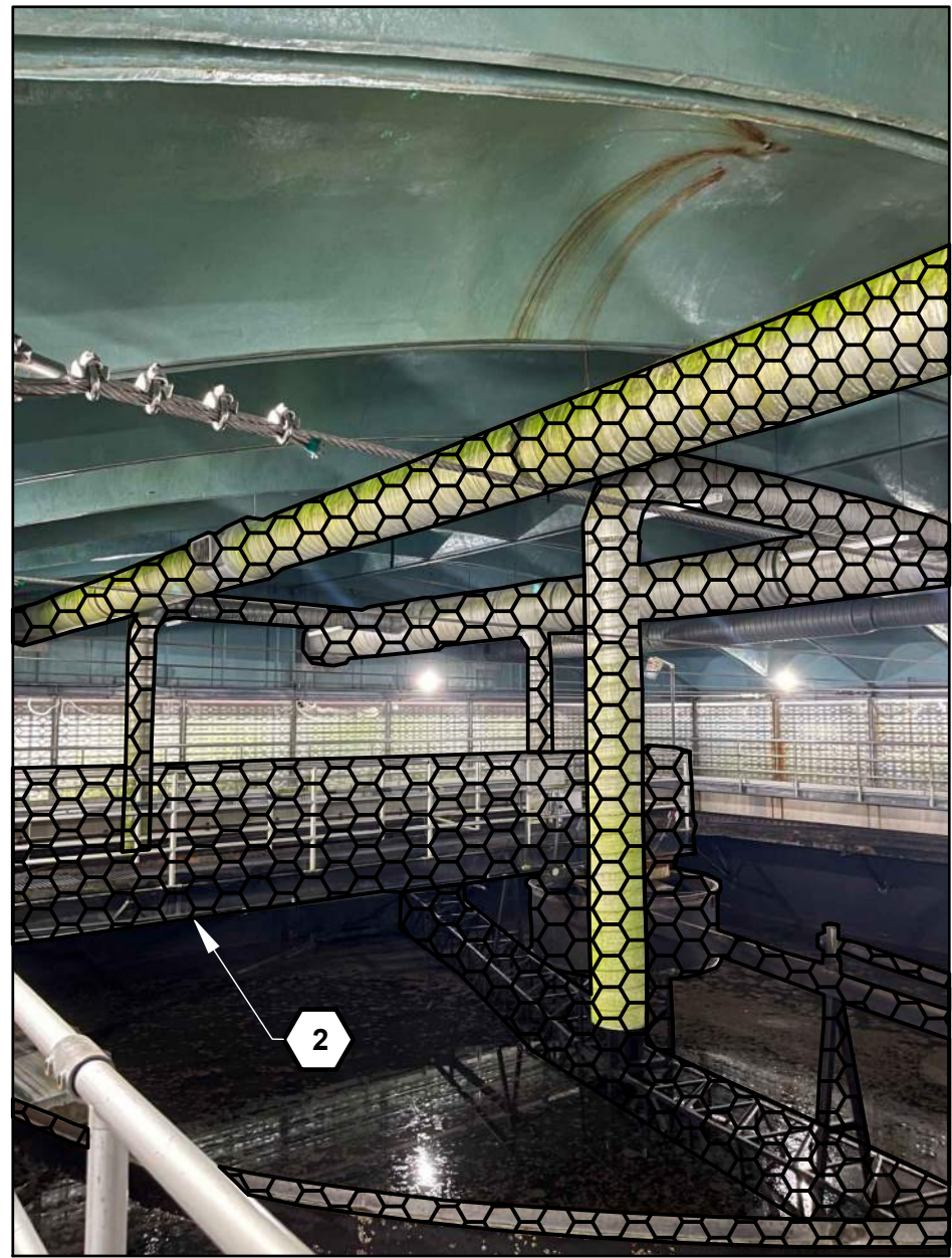
1 SECONDARY CLARIFIER FOUL AIR DUCTING (TYP)
