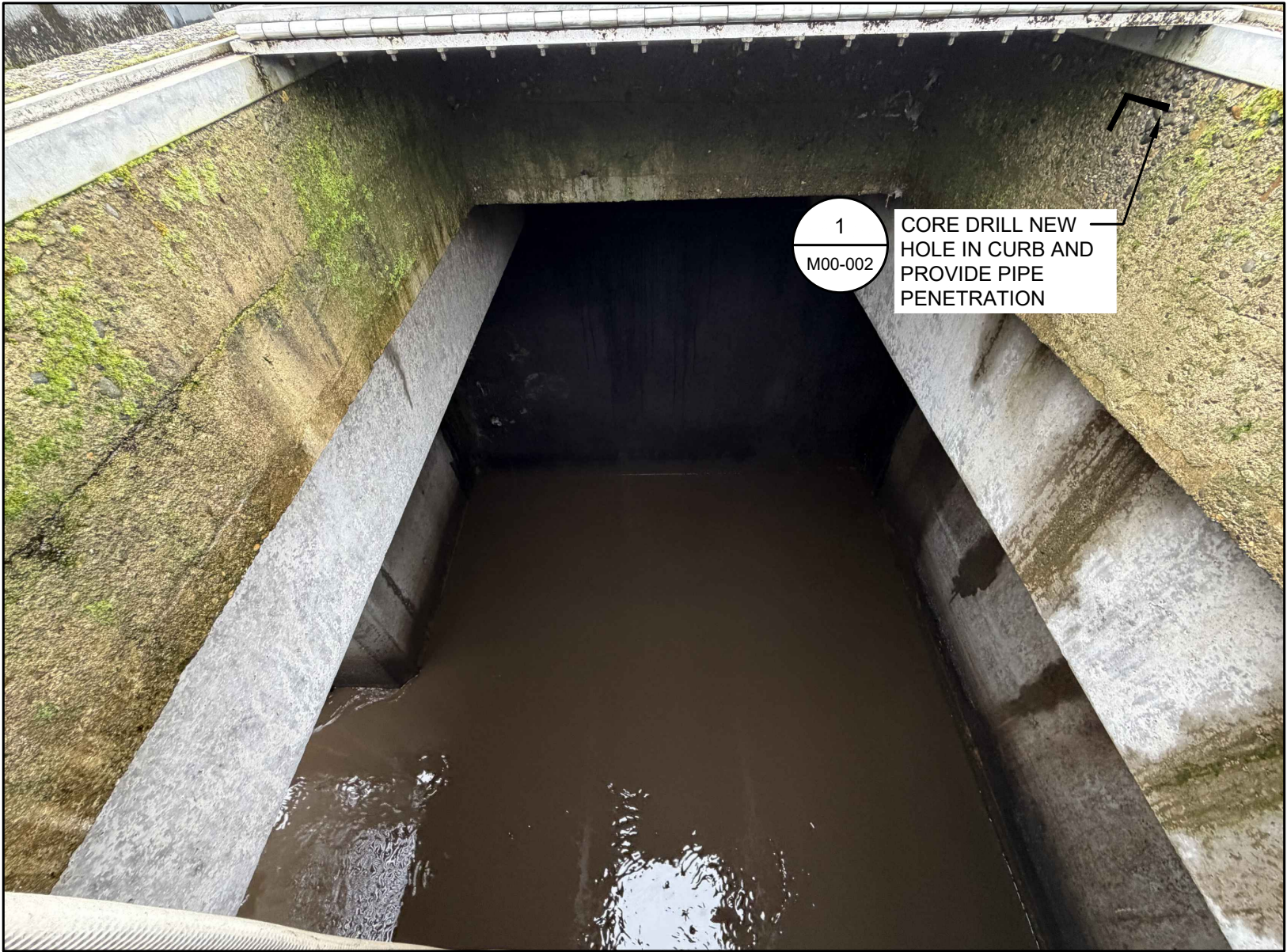
PHOTO 3 SUPPLEMENTAL CARBON PIPING ROUTING
