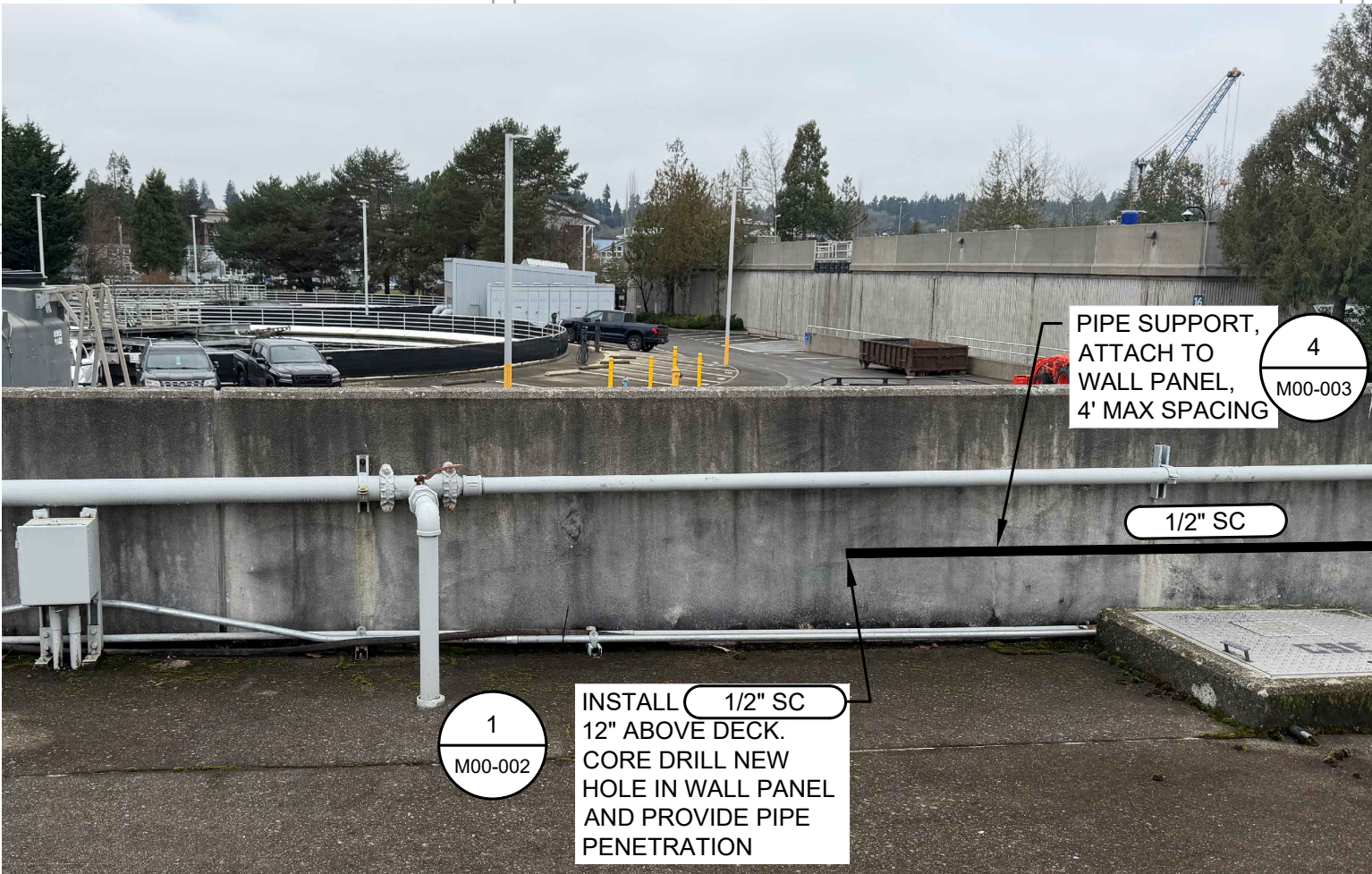
PHOTO 3 SUPPLEMENTAL CARBON PIPE ROUTING
