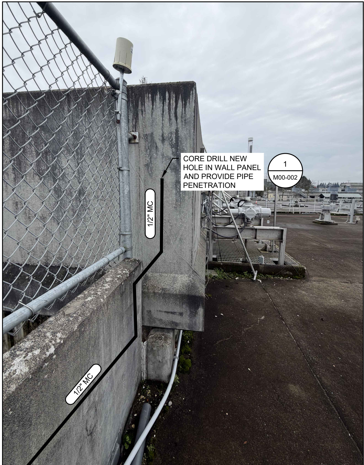
PHOTO 1 SUPPLEMENTAL CARBON PIPING ROUTING
