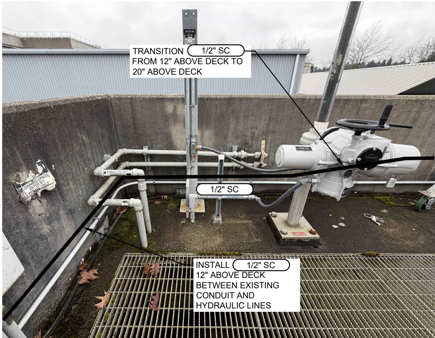
PHOTO 2 SUPPLEMENTAL CARBON PIPE ROUTING
