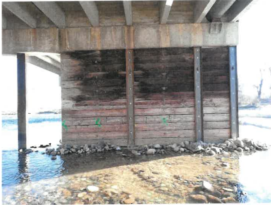
Repair of Timber Piles 3, 5, & 6 at Pier 3 Looking North.
