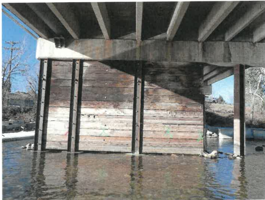
Repair of Timber Piles 3, 5, & 6 at Pier 3 Looking South.
