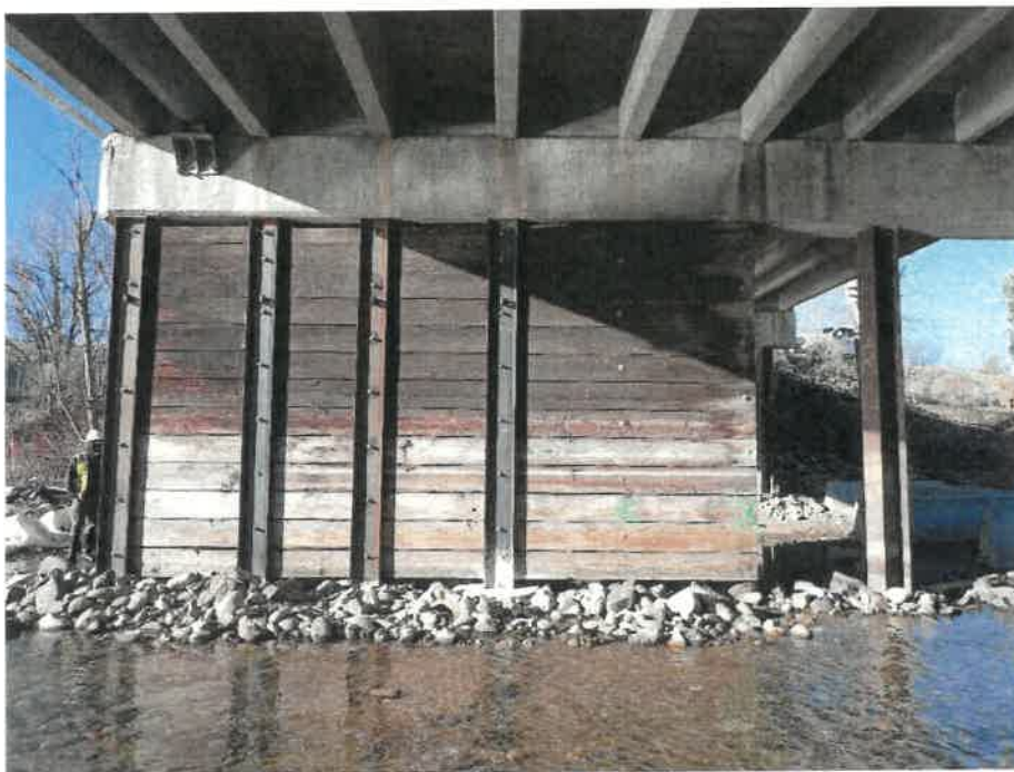
Repair of Timber Piles 4-6 at Pier 2 Looking South.
