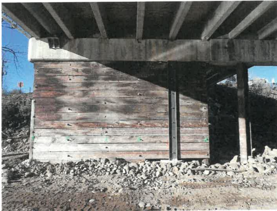
Repair of Timber Pile 2 at Pier 1 Looking South.
