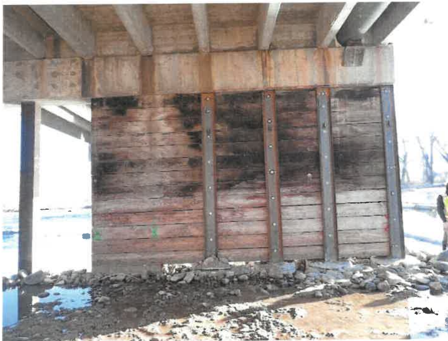
Repair of Timber Piles 4-6 at Pier 2 Looking North.
