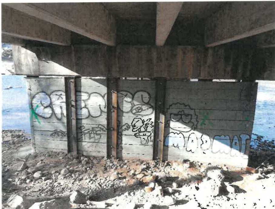
Repair of Timber Piles 3-5 at Pier 8 Looking South.
