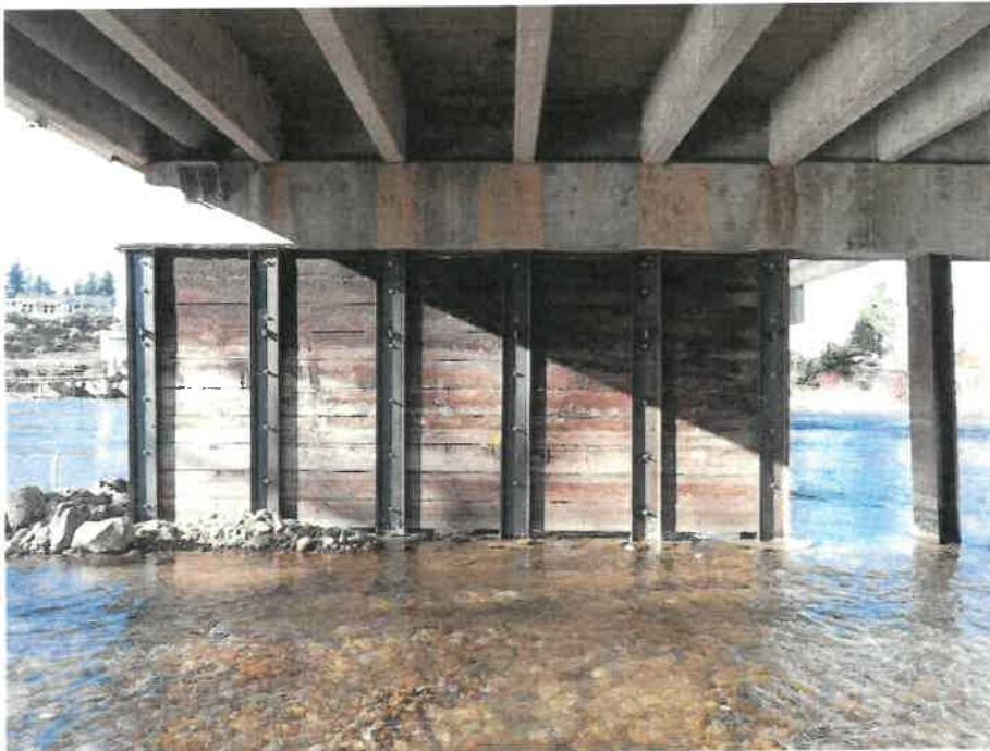
Repair of All Timber Piles at Pier 7 Looking South.
