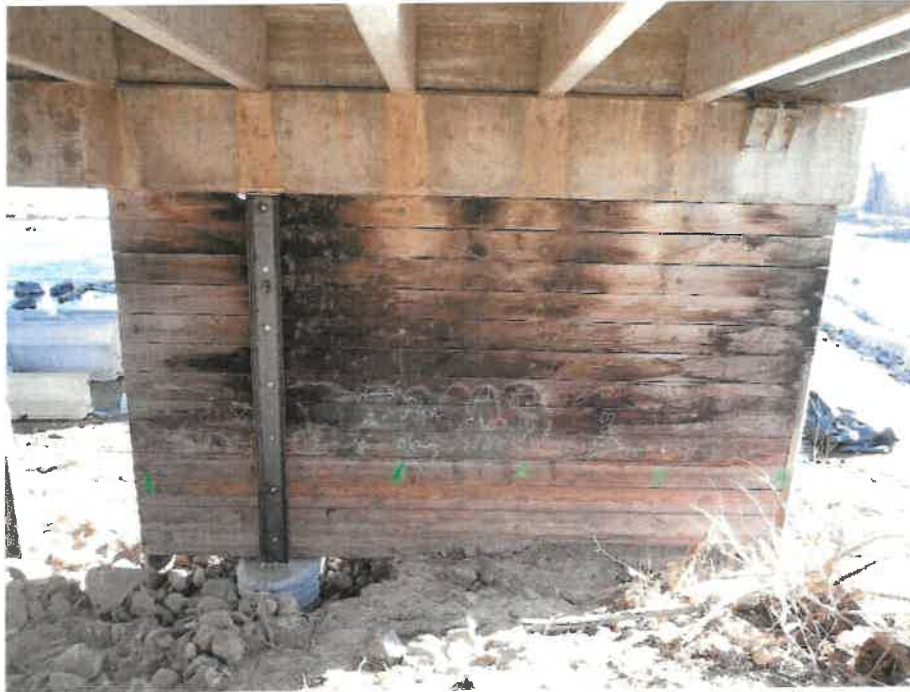
Repair of Timber Pile 2 at Pier 1 Looking North.
