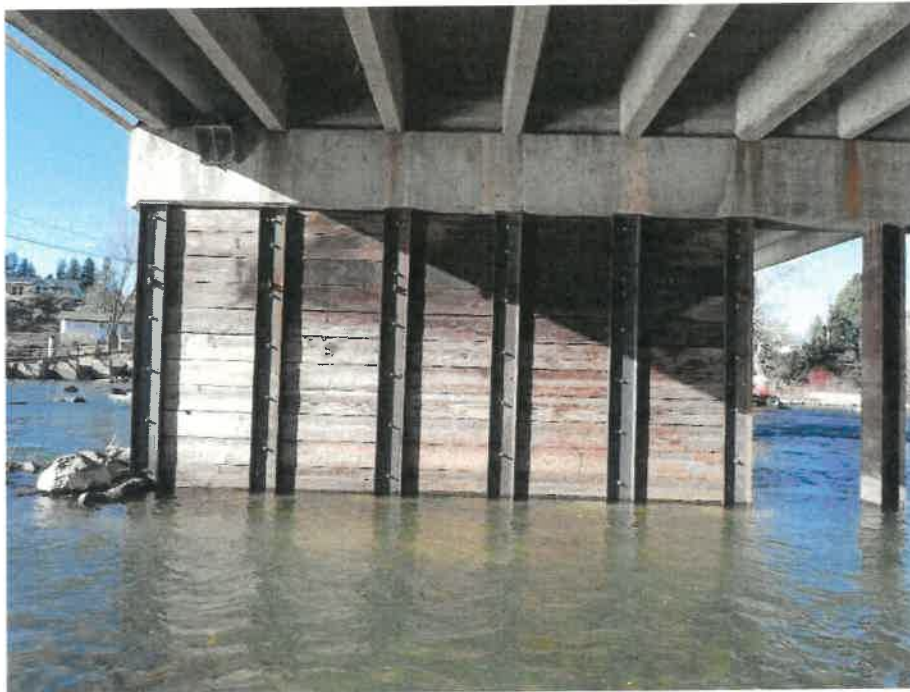
Repair of All Timber Piles at Pier 6 Looking South.
