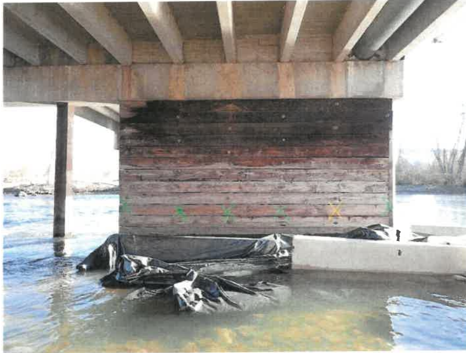
Pier 5 Looking North.
