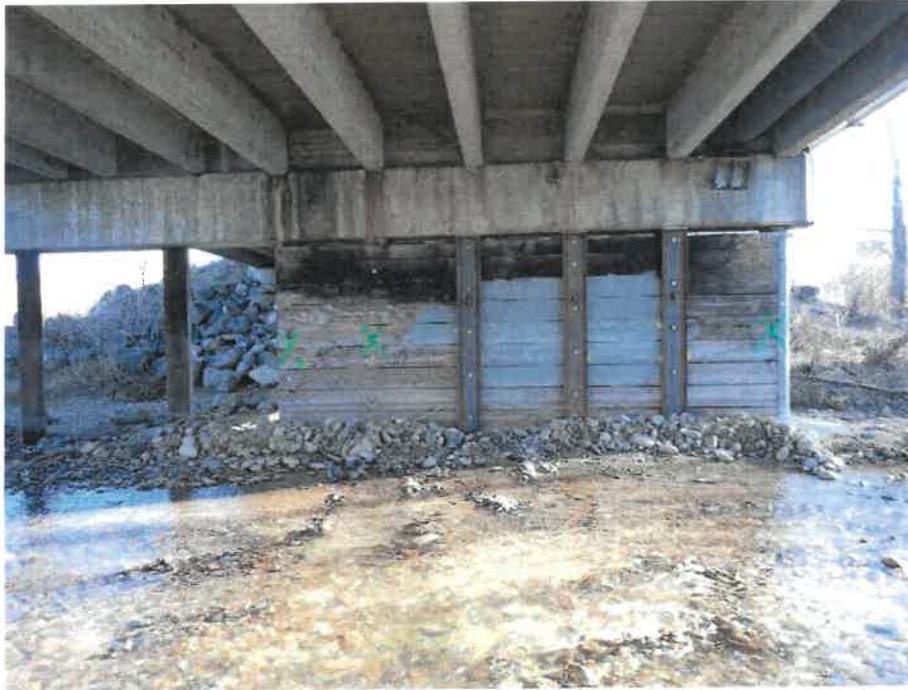
Repair of Timber Piles 3-5 at Pier 8 Looking North.
