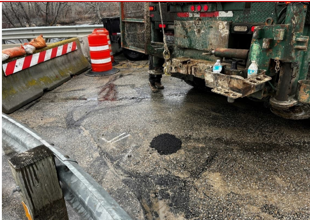
B-2, after completion of drilling operations
