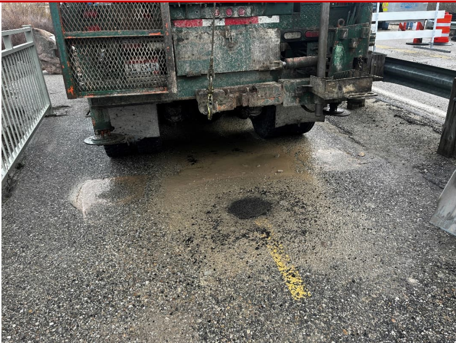
B-6, after completion of drilling operations
