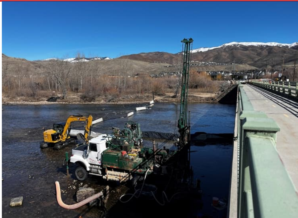
B-3, prior to completion of drilling operations
