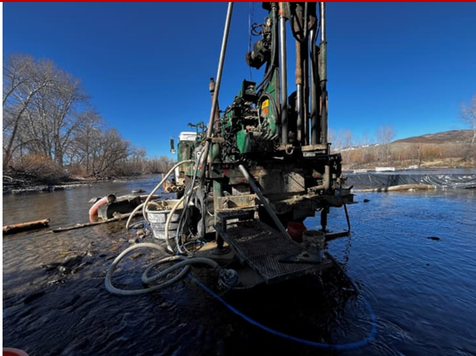
B-3, prior to completion of drilling operations
