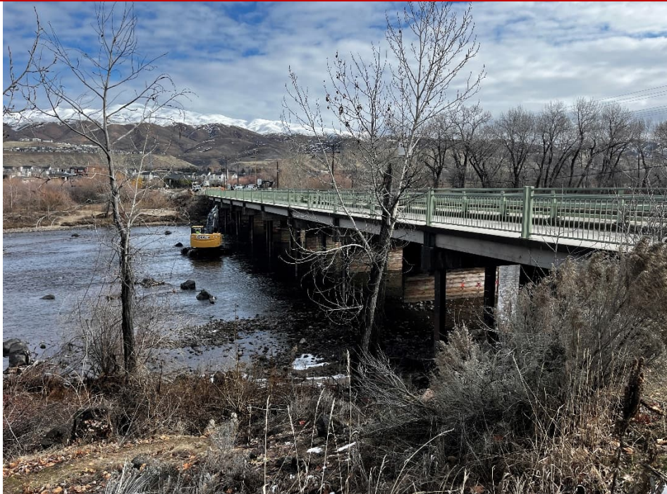
Looking northeast towards B-3, B-4, B-5
