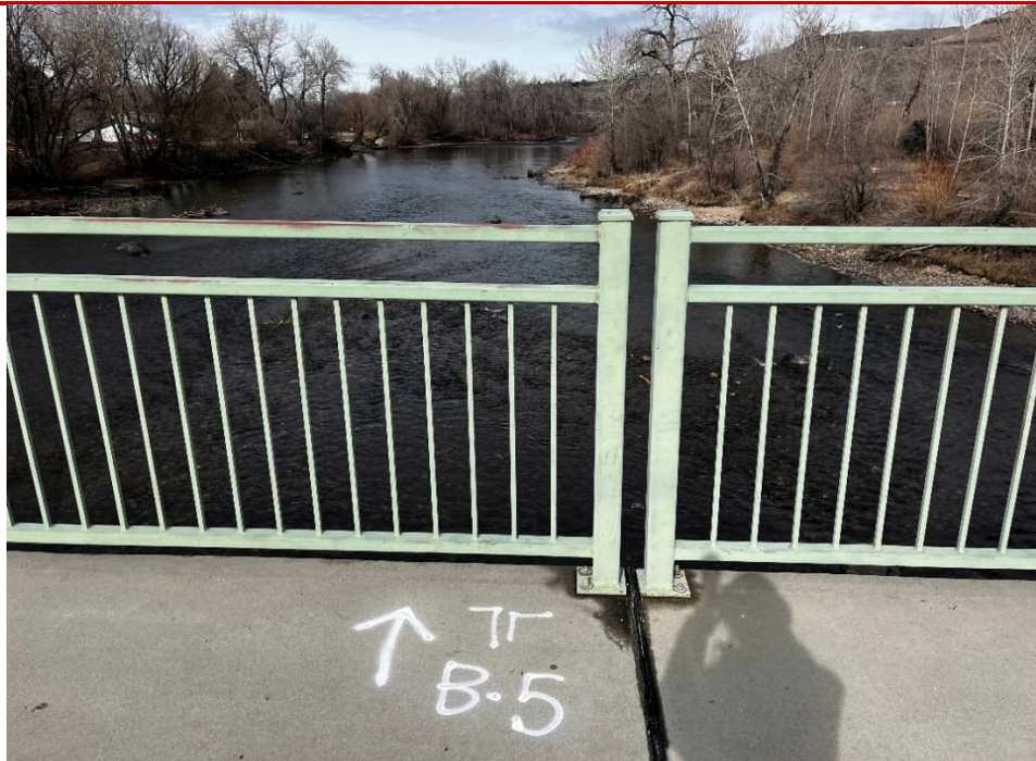
Looking northwest towards B-5
