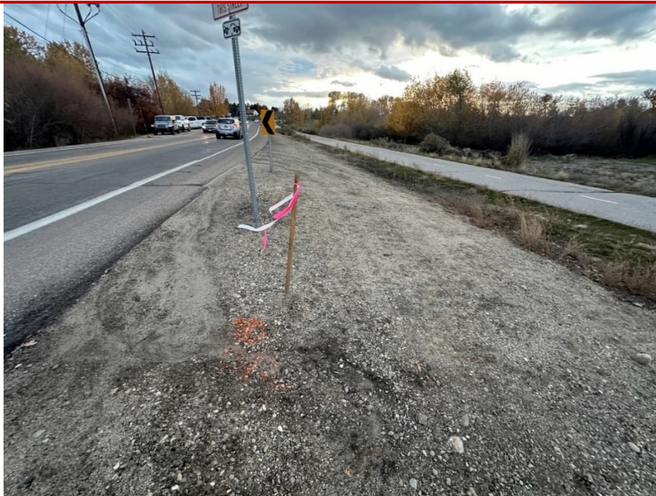
RW-16, prior to completion of drilling activities
