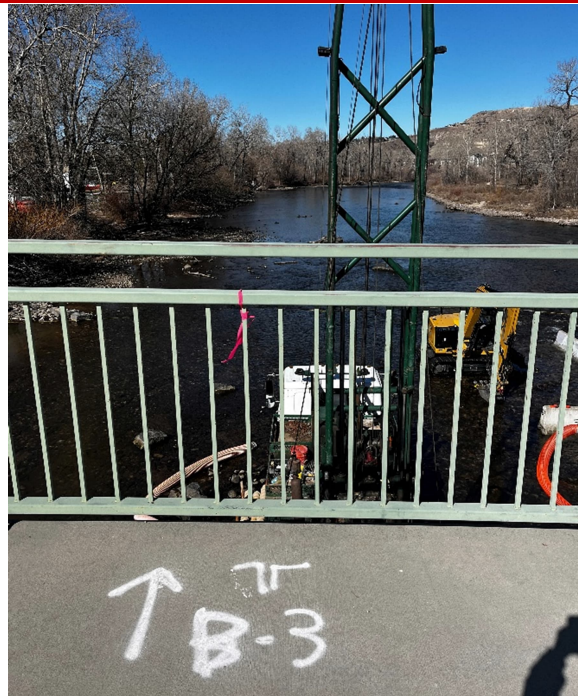
Looking northwest towards B-3
