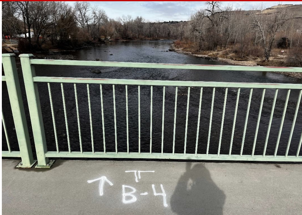
Looking northwest towards B-4
