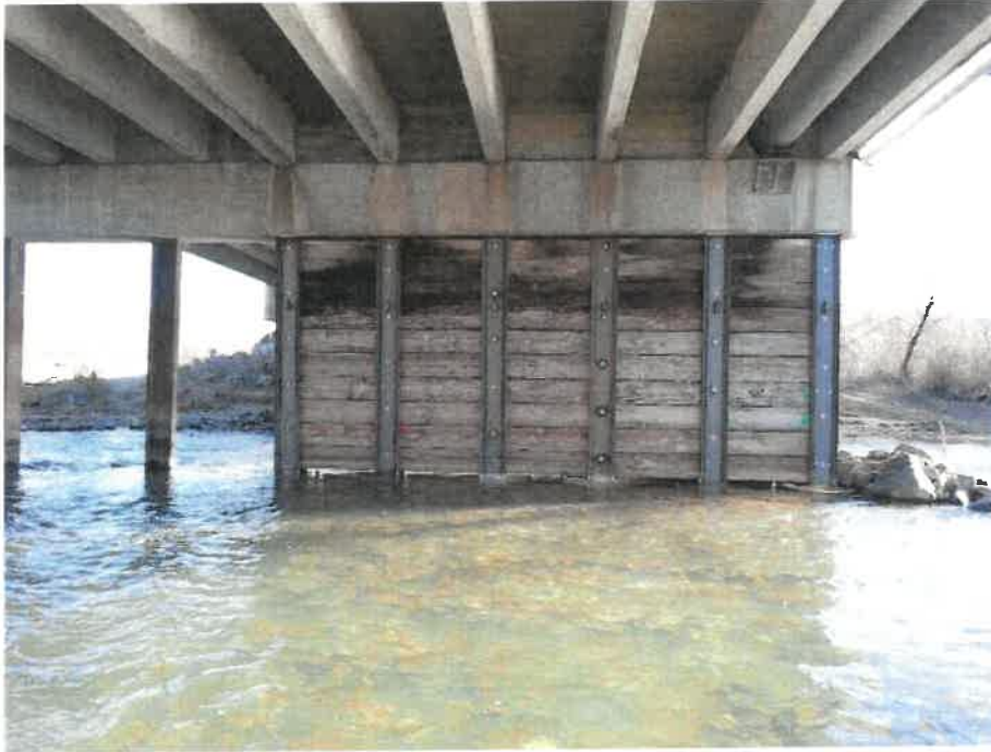
Repair of All Timber Piles at Pier 7 Looking North.
