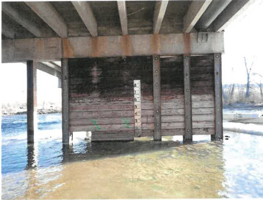
Repair of Timber Piles 1 & 4-6 at Pier 4 Looking North.
