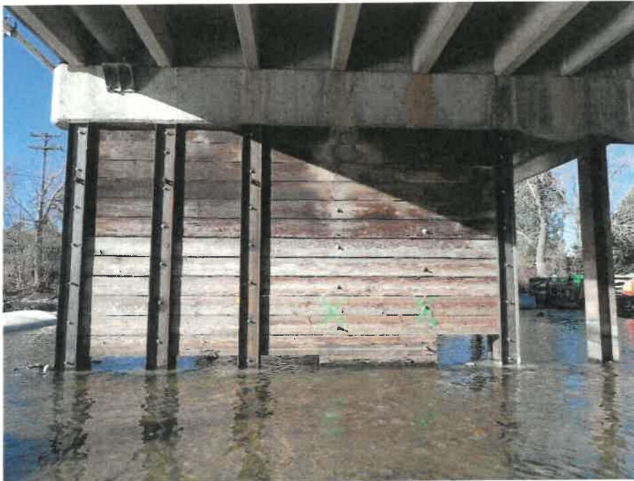
Repair of Timber Piles 1 & 4-6 at Pier 4 Looking South.
