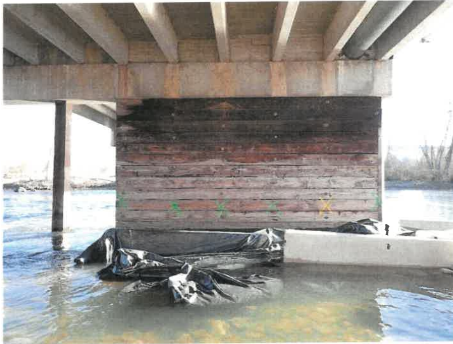
Pier 5 Looking North.
