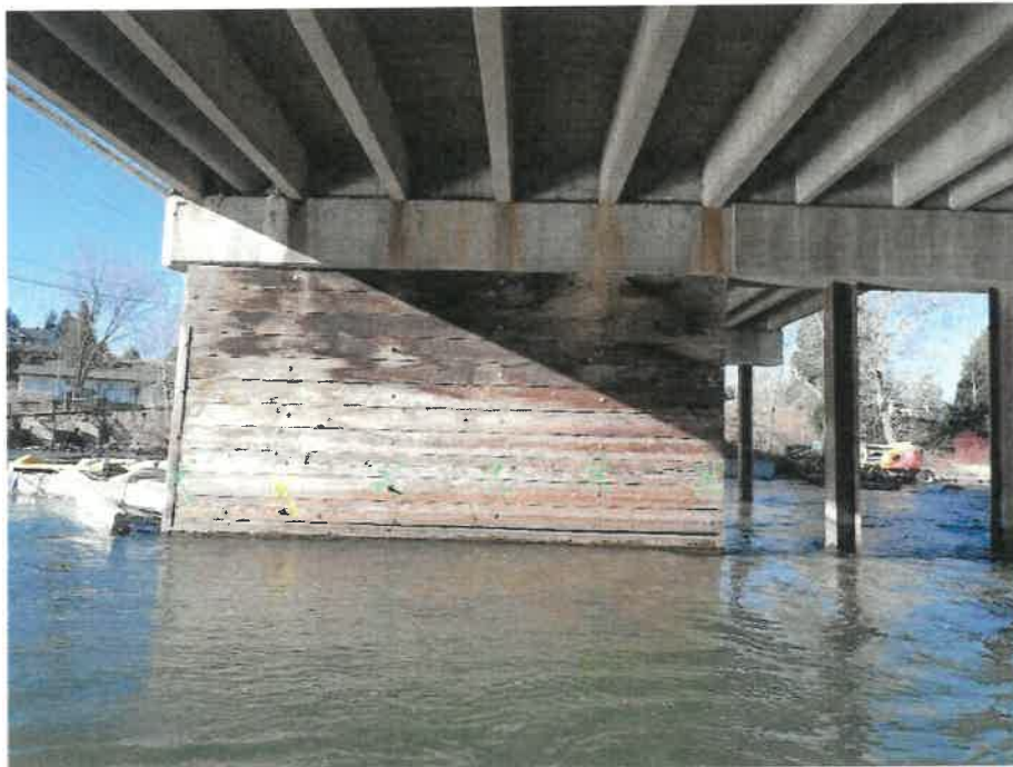
Pier 5 Looking South.
