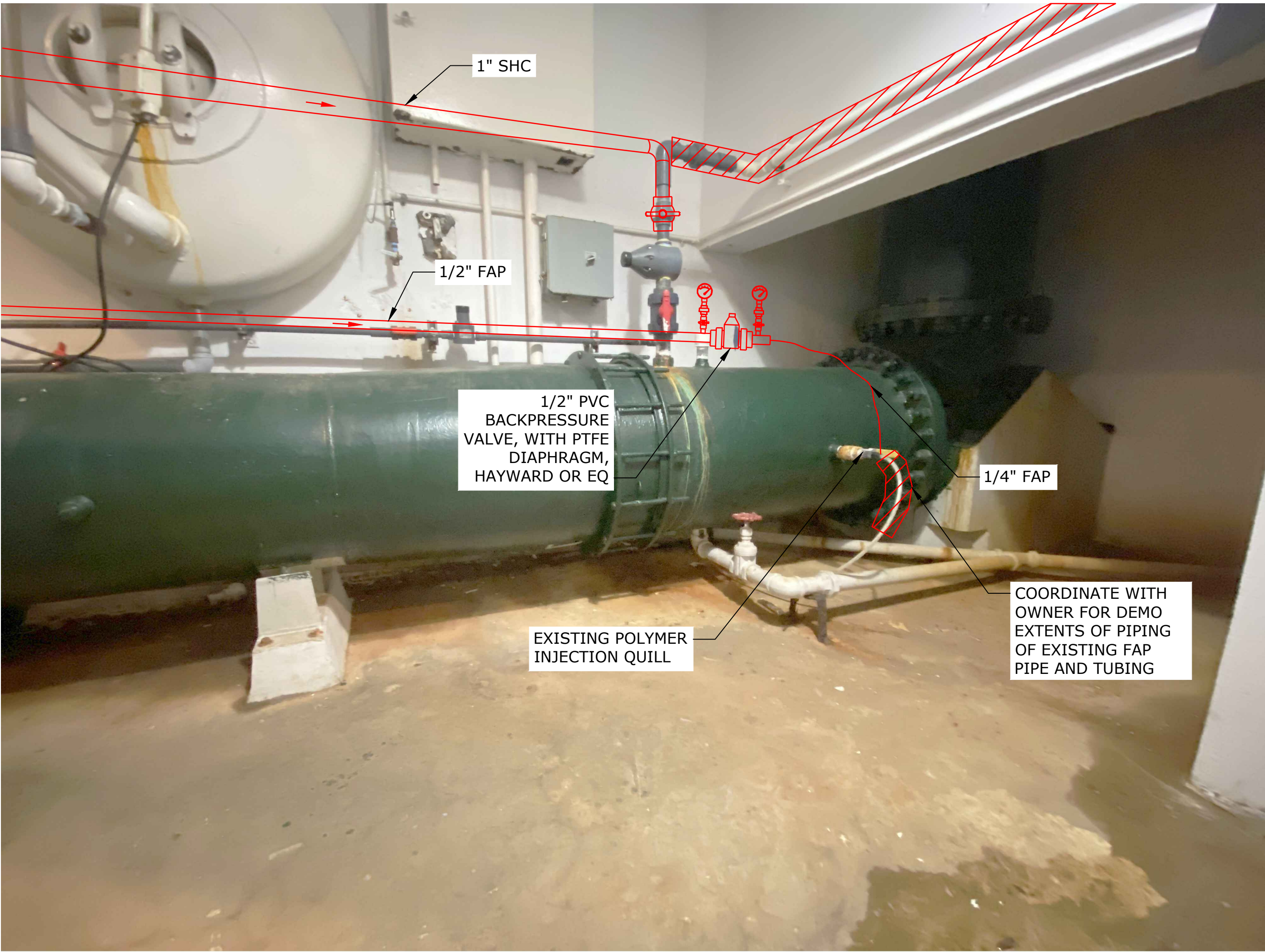
POLYMER PIPE ROUTING DETAIL
