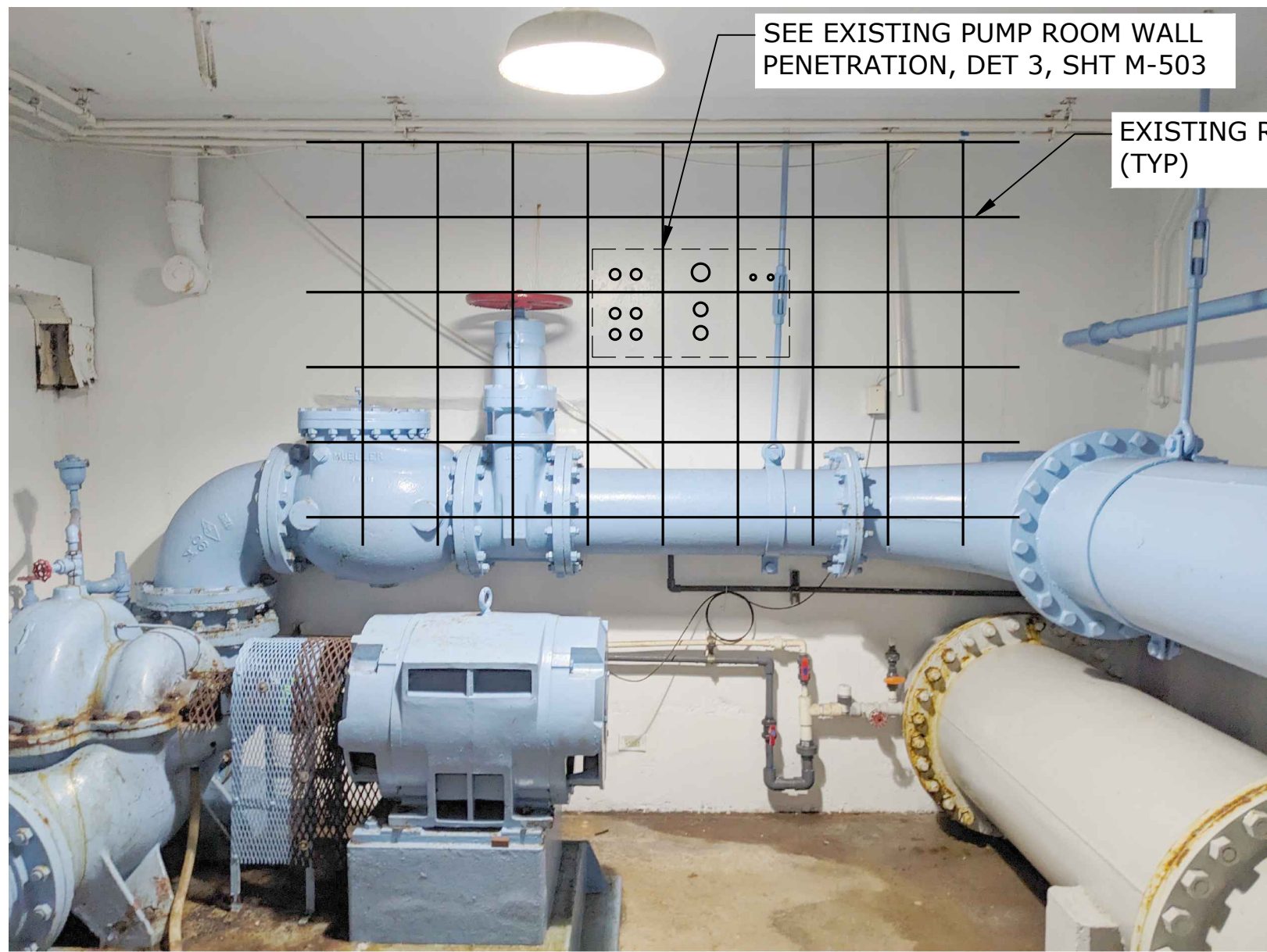
EXISTING PUMP ROOM WALL PENETRATION DETAIL
