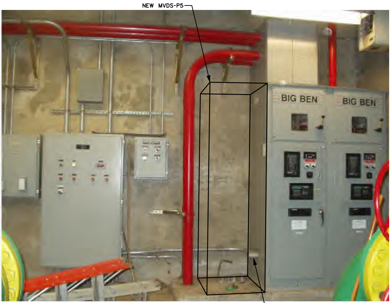
SOUTH WEST WALL ELECTRICAL DEMOLITION
