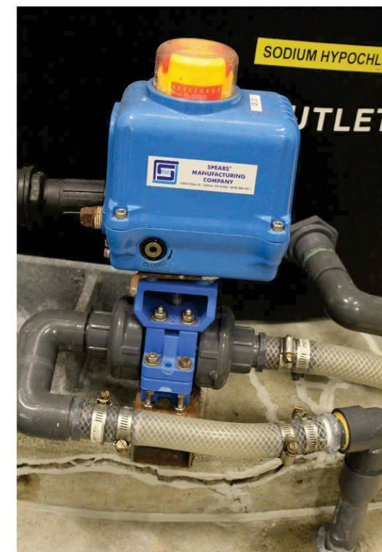
2 HYPO TANK MOV REFERENCE IMAGE (E)
