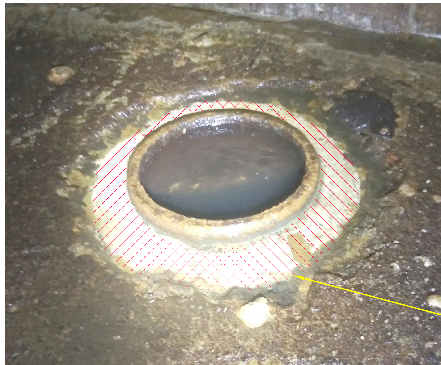
4 R1-1 NTS PHOTO DETAIL INLET/OUTLET PIPE
