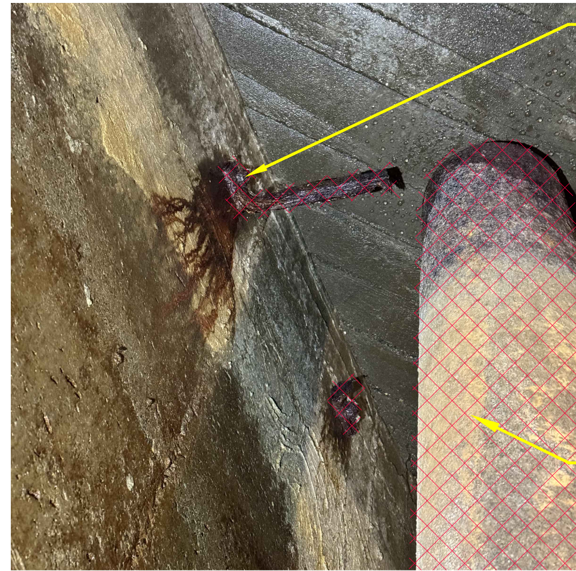
1 R1-1 NTS PHOTO DETAIL - OVERFLOW PIPE TOP OF OVERFLOW PIPE AND SUPPORT
