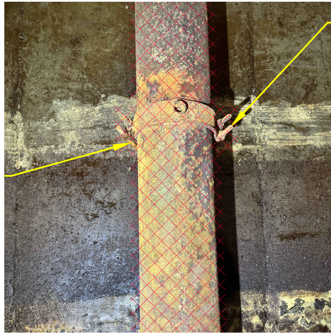
2 R1-1 NTS PHOTO DETAIL - OVERFLOW PIPE MIDDLE OF OVERFLOW PIPE AND SUPPORT
