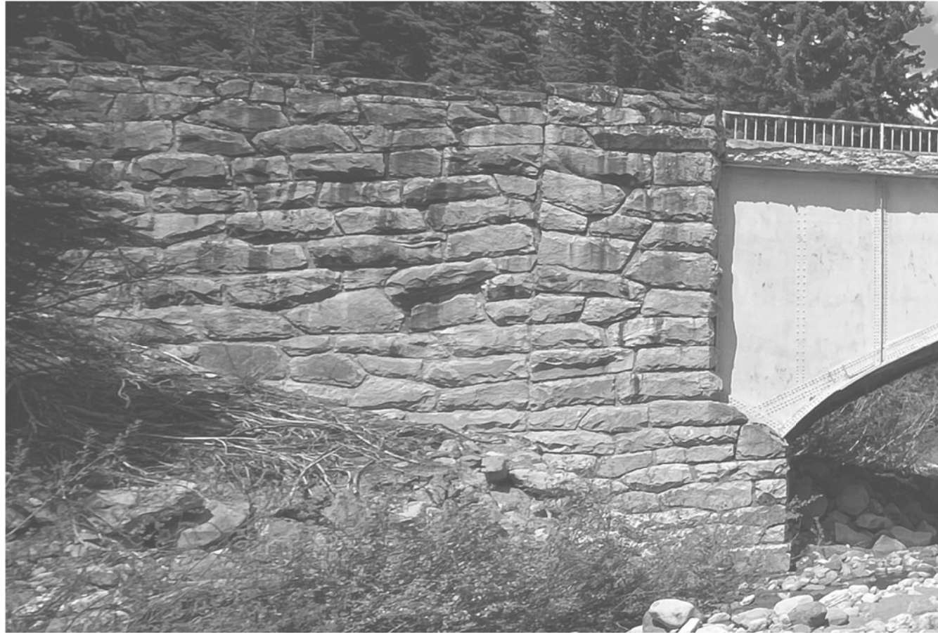
STONE PATTERN AT EXISTING FRYINGPAN CREEK BRIDGE
