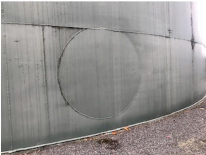
View of lower shell, past access panel.
