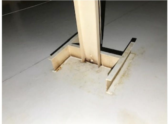
View of interior column base – typical.
