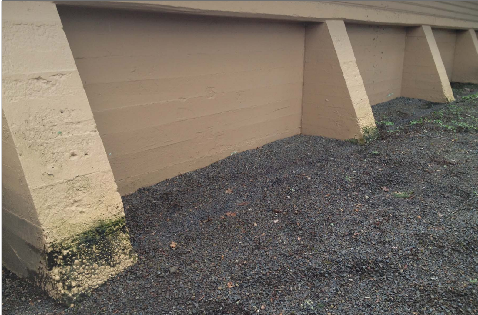
Photo 1: 1MG Reservoir, Northeast Corner
