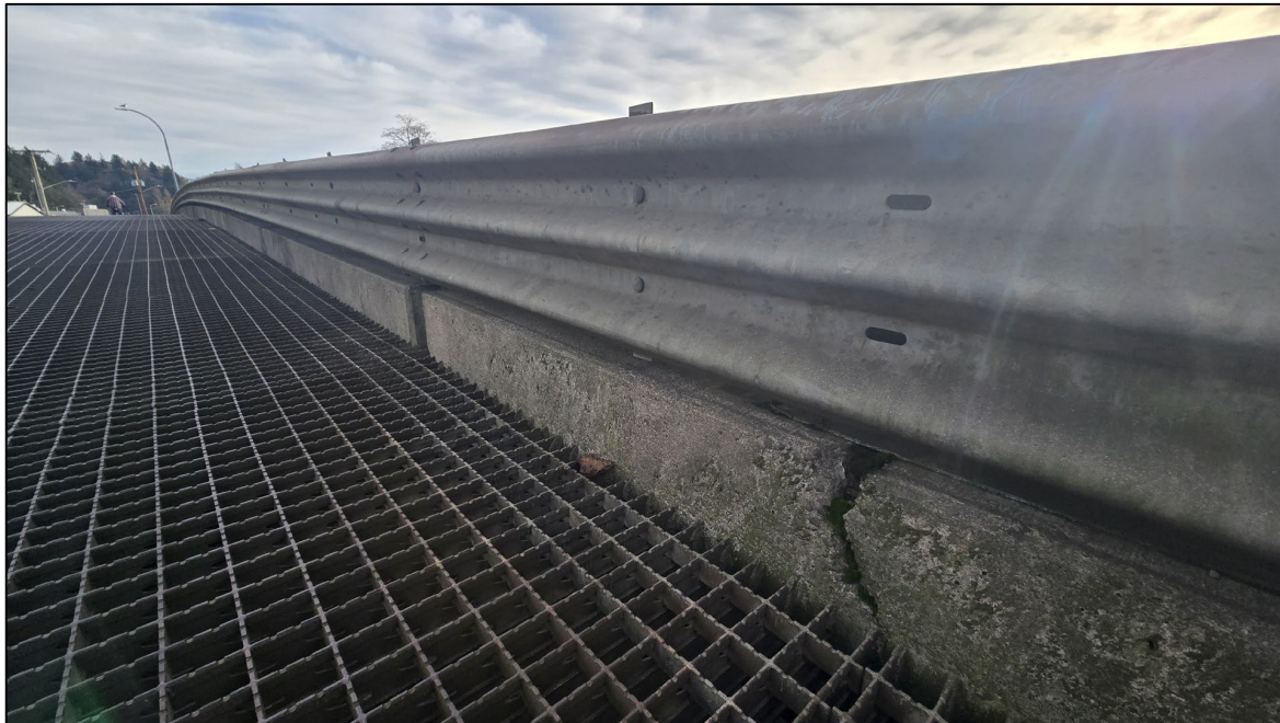
Photograph 2. View of homogenous concrete blocks to be replaced.
