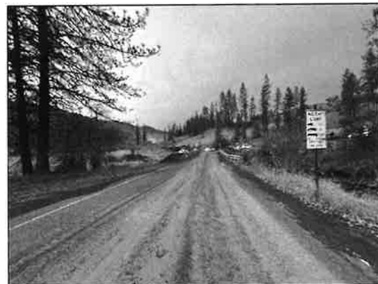
Photograph 4. Site photograph taken from Clear Creek Road south of the bridge, looking northwest toward the bridge.
