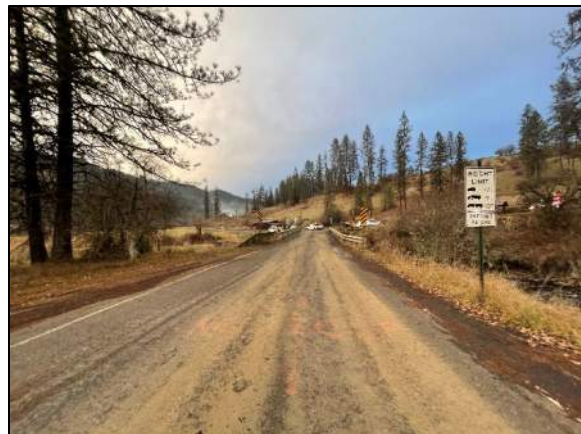
Photograph 4. Site photograph taken from Clear Creek Road south of the bridge, looking northwest toward the bridge.
