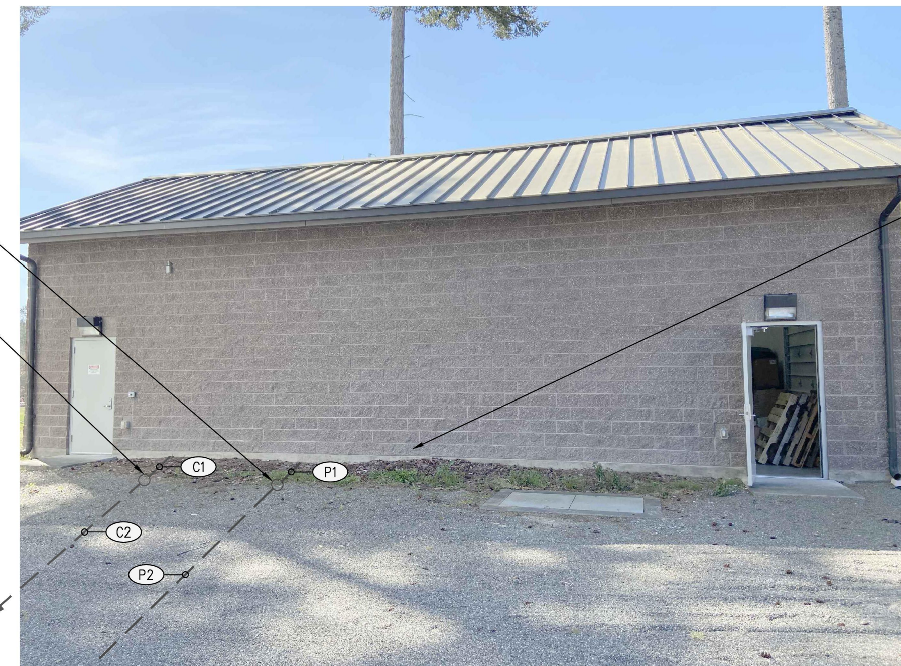
BPS EXTERIOR - EXISTING CONDUIT LOCATIONS NO SCALE
