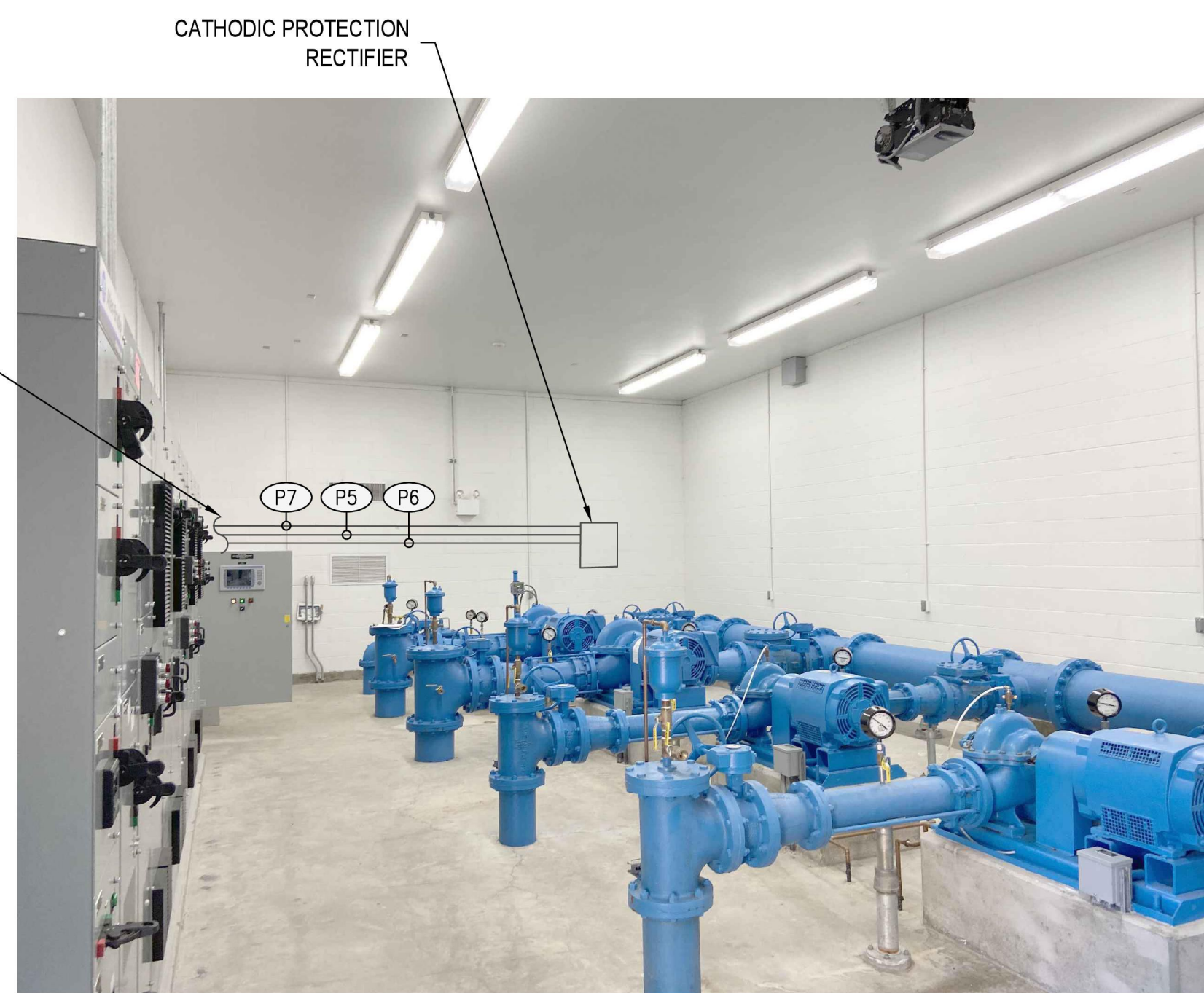
CATHODIC PROTECTION RECTIFIER NO SCALE
