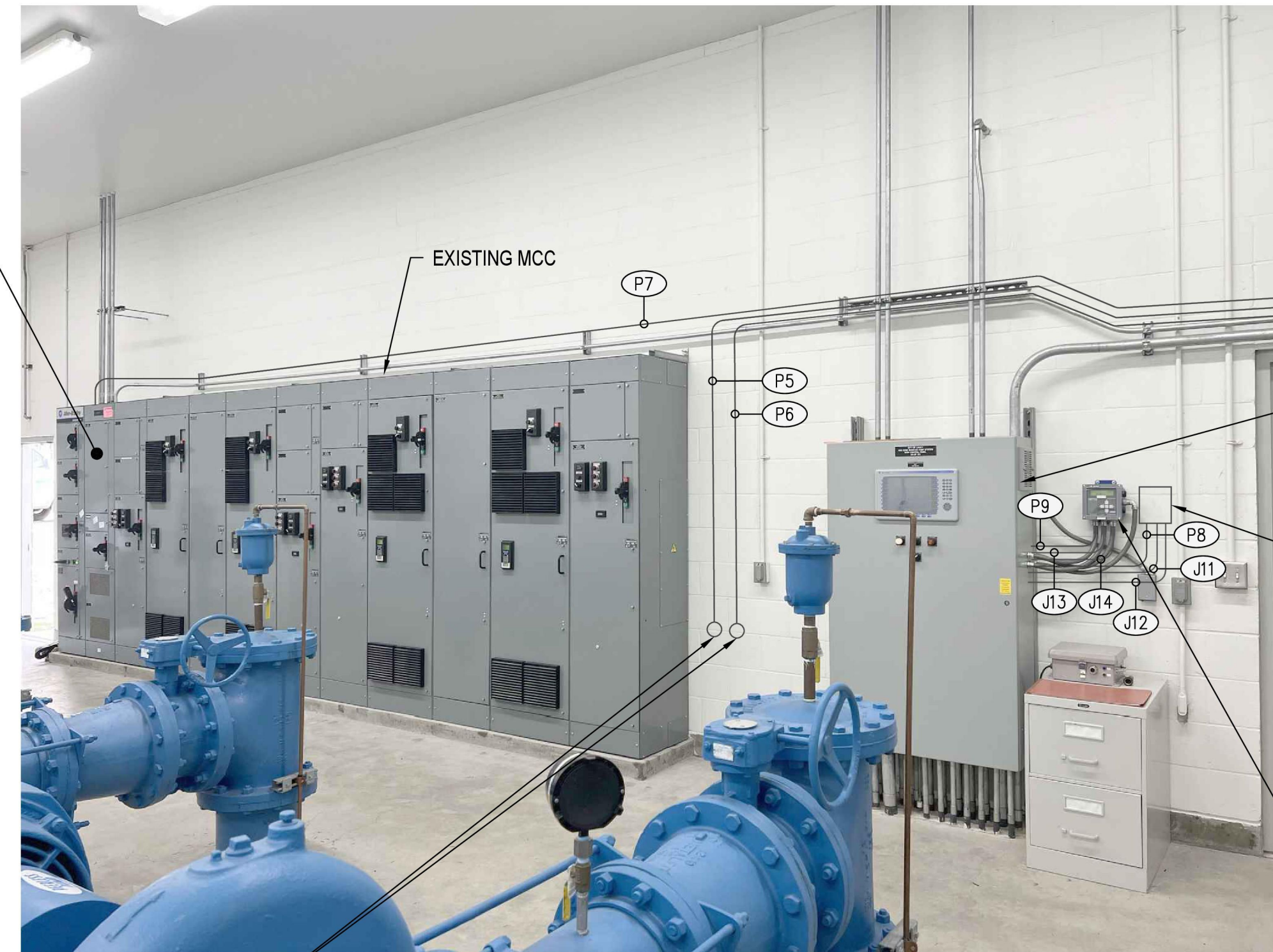
BPS INTERIOR - CONDUIT ROUTING NO SCALE
