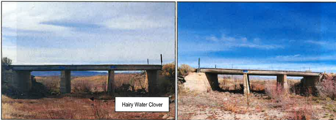
Figure 6. 23795 bridge, downstream (left) and upstream (right) bridge faces (FA Survey, 2023)
