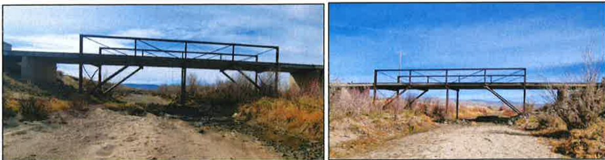
Figure 5. 23800 bridge, downstream (left) and upstream (right) bridge faces (FA Survey, 2023)
