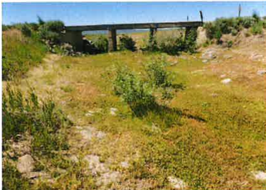
Photo 1: Wetland A, downstream of Bridge 23795 (June 24, 2024)
