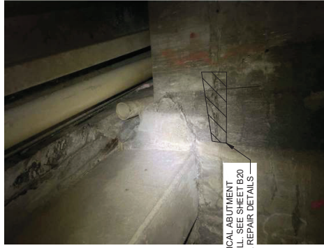
TYPICAL ABUTMENT SPALL REPAIR
