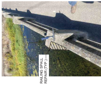
TYPICAL BARRIER POST SPALL REPAIR N.T.S.
