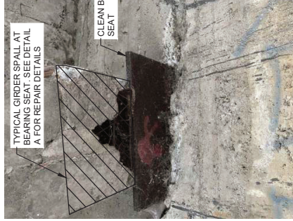
REMOVE AND REPAIR ALL LOOSE CONCRETE. CLEAN EXPOSED REINFORCEMENT. SEE SHEET B20
