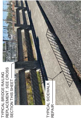
TYPICAL SIDEWALK AND RAIL REPAIRS N.T.S.
