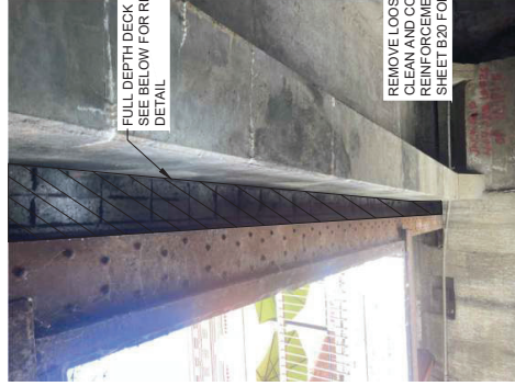
FULL DEPTH DECK REPAIR
