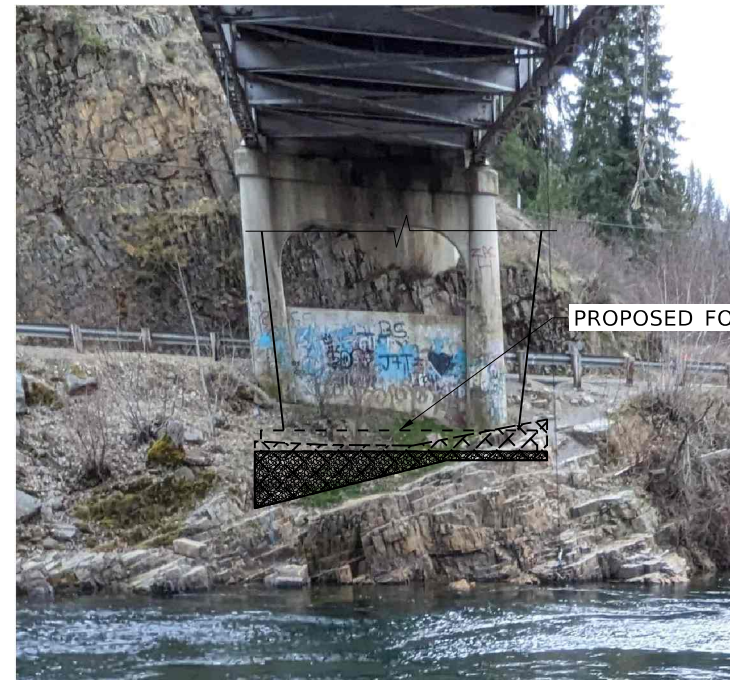
PIER 1 (LOOKING EAST)
